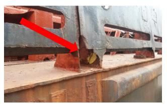
Engine room skylights frames bent and corroded through.
