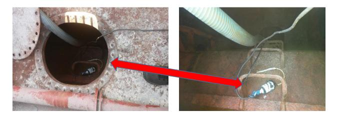
Ballast tanks manholes covers not tight due to bolts wastage.
