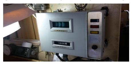
Emergency equipment for 2-way communication batteries missing.
