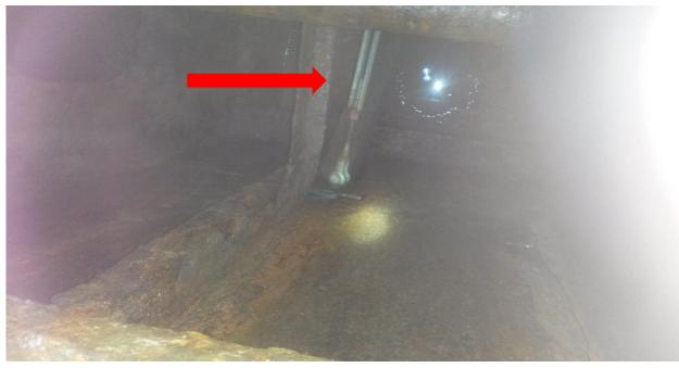
Ballast system out of order. Ballast water pumped out by submersible pump, unsafe electrical power supply.
