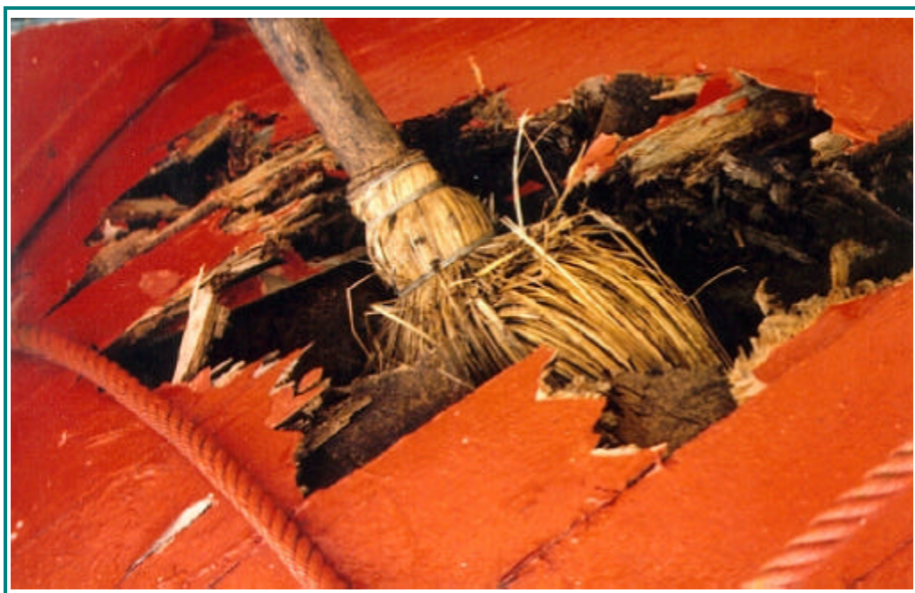
Deteriorated skin of a (wooden!) lifeboat, which leaves no room for speculations on the availability of this vital lifesaving appliance.
