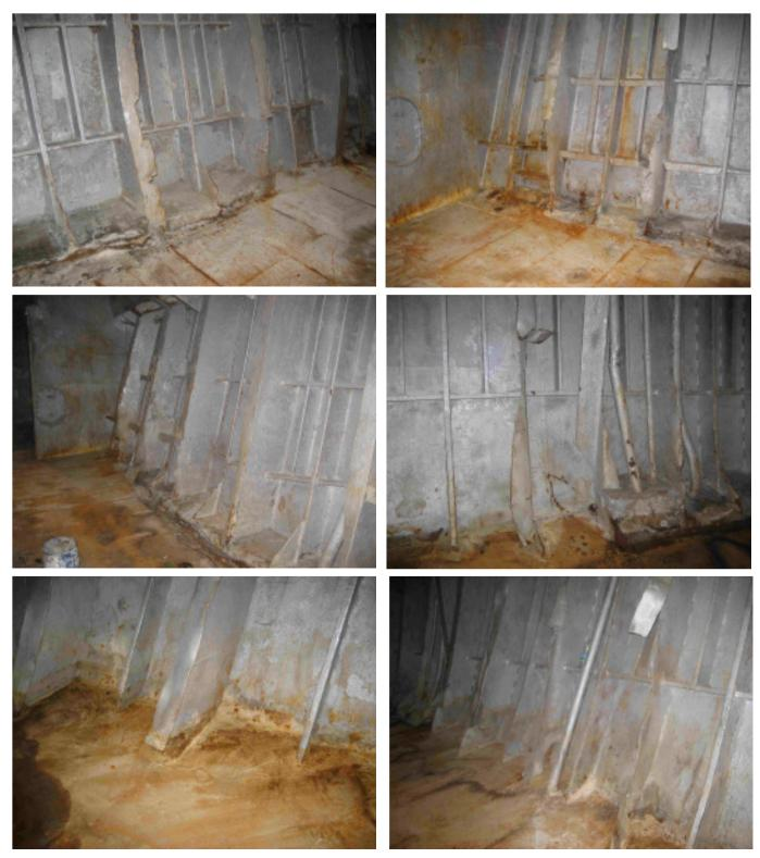
After that several temporary repairs are carried out before departure and all nonstructural deficiencies are rectified in the detention port, a single voyage is agreed by PSC Authority to the owner and Administration towards the indicated repair yard.
