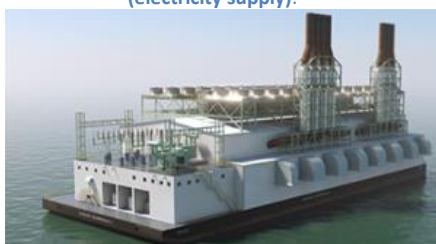
Figure 4.10 – LNG fuelled floating power plant
