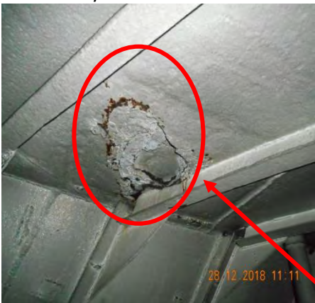
Penetrations of the superstructure by air condition piping system without any authorization
