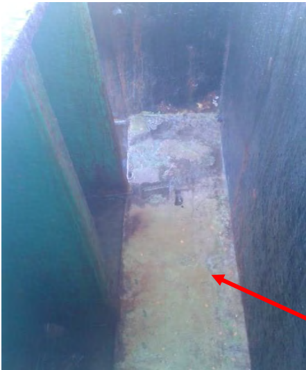
Vertical bulk head, with holes around piping penetrations
