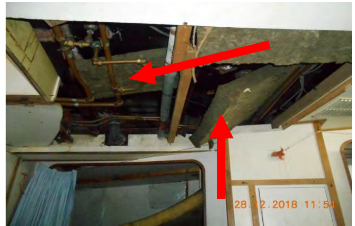
The condition of the roof of the crew cabin. The piping system above the roof insulation
