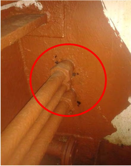
Vertical bulk head, with holes around piping penetrations
