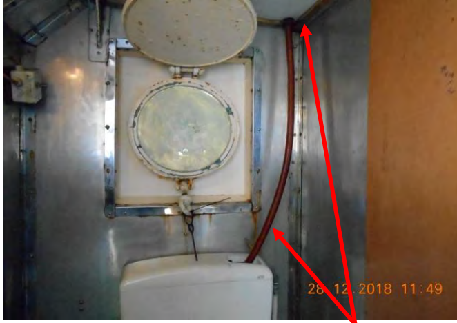
The way of providing water to the toilet
