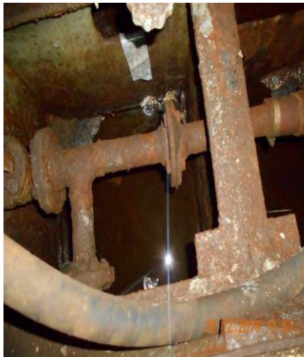
The Steering Gear hydraulic piping system
