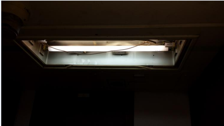
Portable electrical cable not safe; Neon light protection missing.
