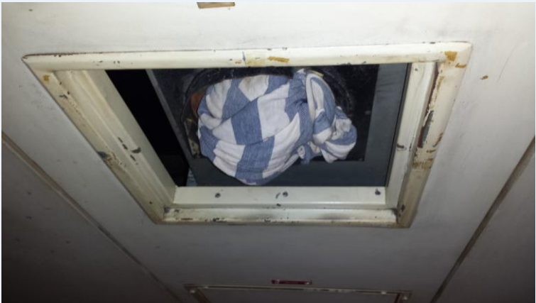
Rags used for closing ventilation.
