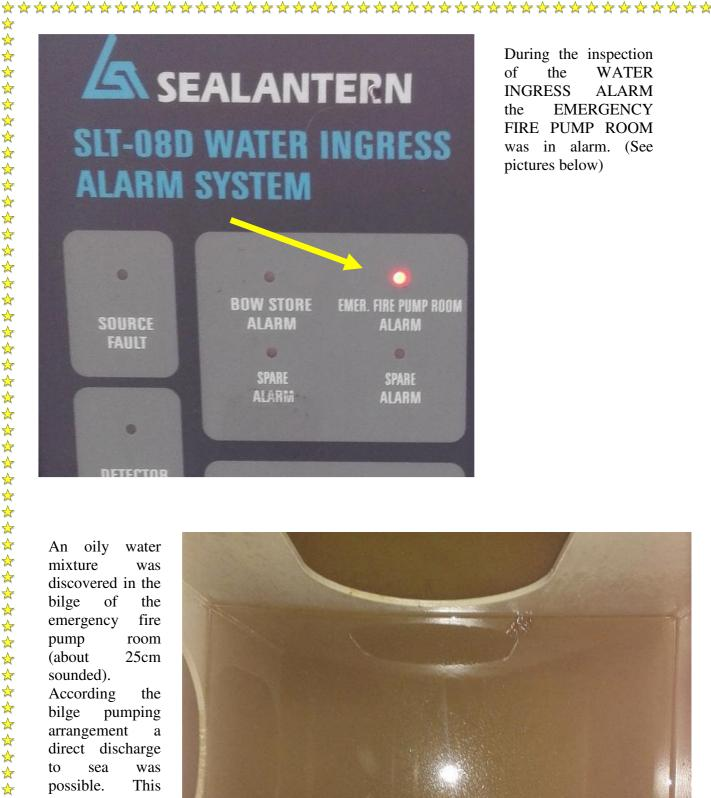
During the inspection the WATER **INGRESS ALARM EMERGENCY** the FIRE PUMP ROOM was in alarm. (See pictures below)
