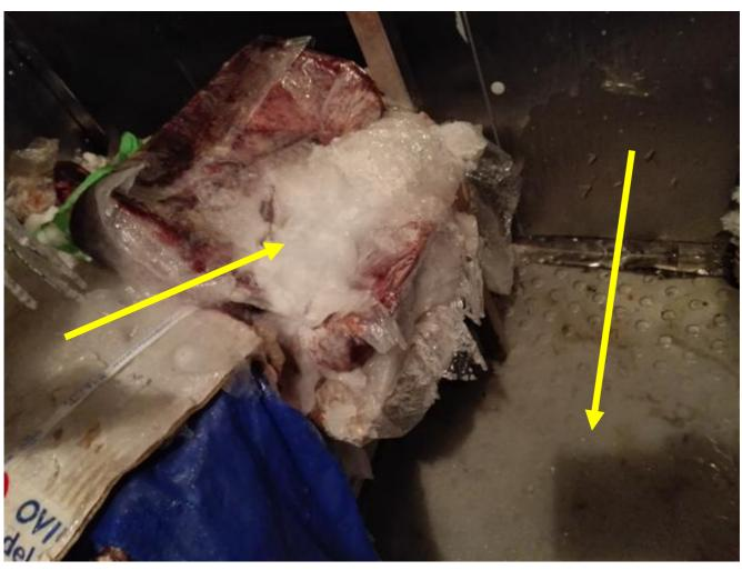
In deep freezer room heavy icing of meat and floor caused by overheating (-10°) and improper gaskets.
