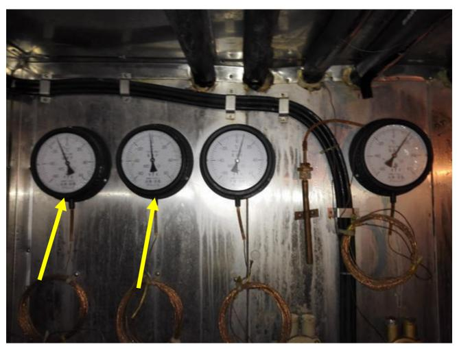
Temperature sensors of freezers fully out of range, resulting in iced meat and rotten food full of mould.
