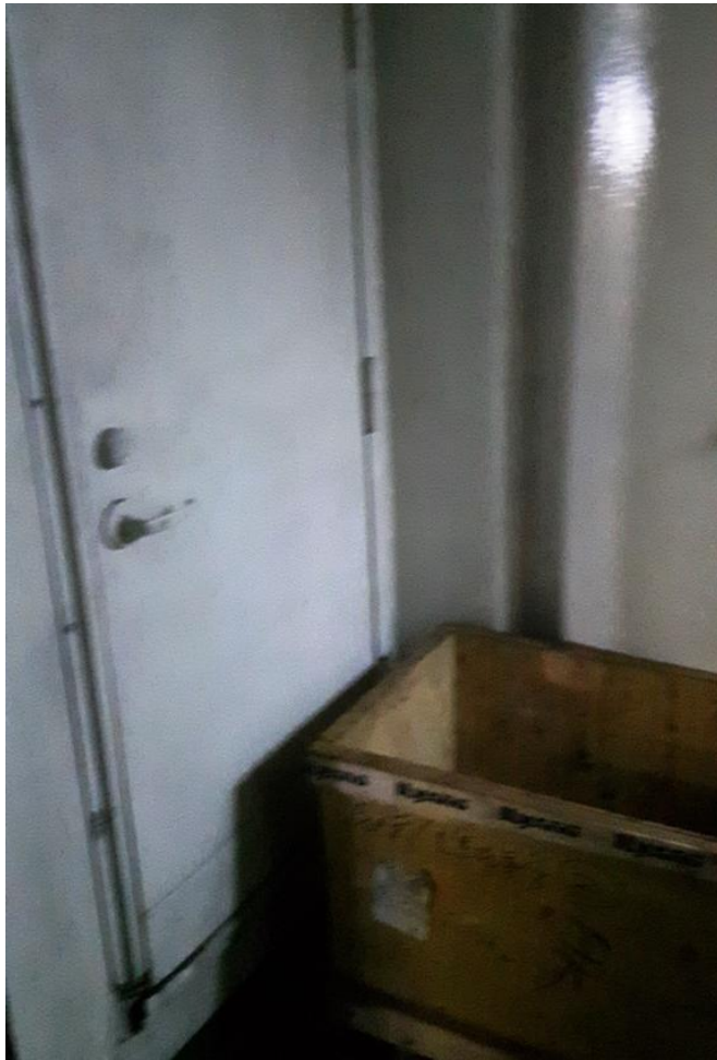
Escape route in galley blocked
