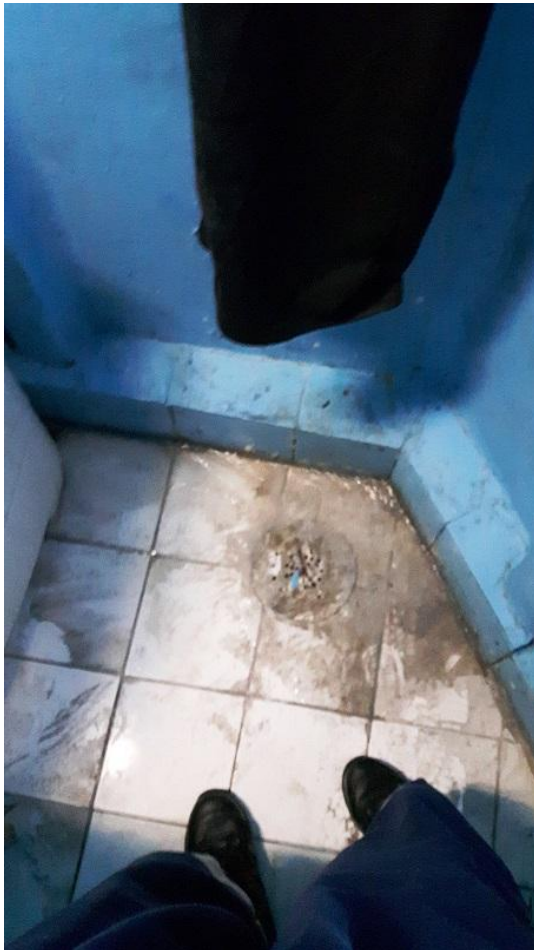
Drainage obstructed
